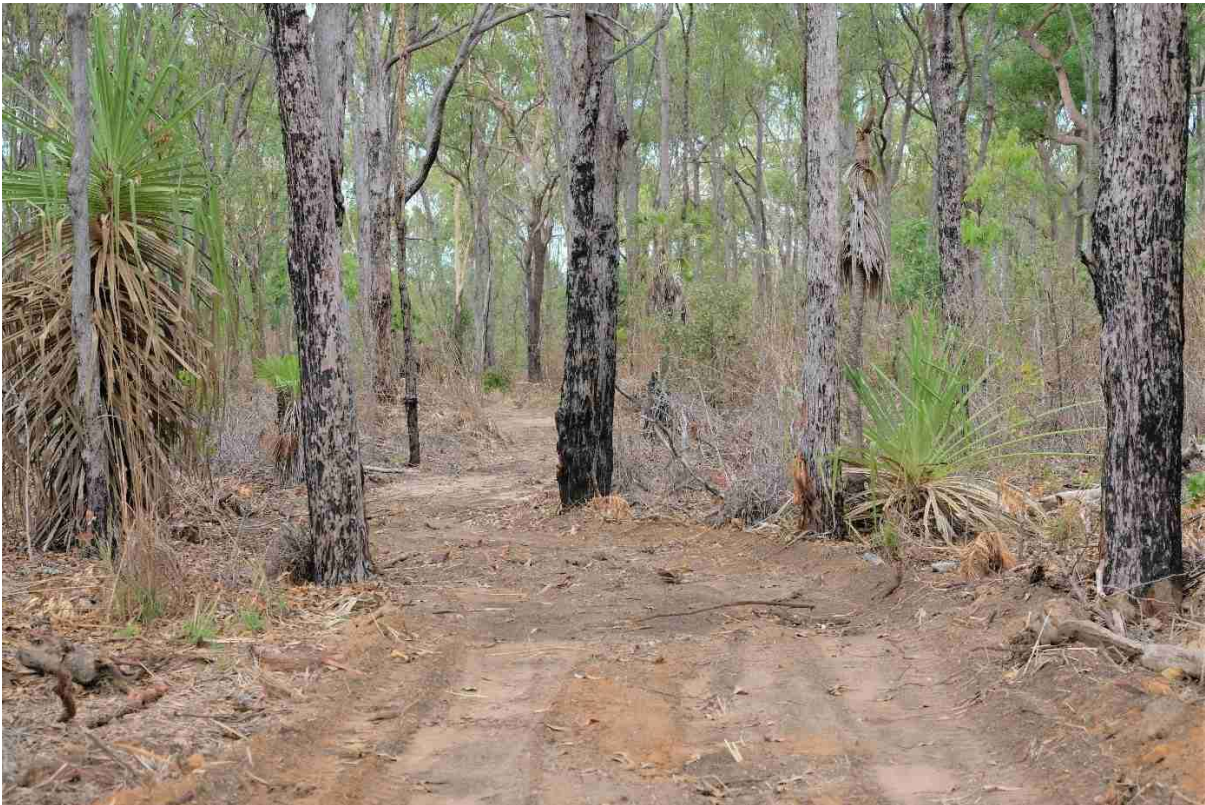
A new "firebreak" in Stage 2
