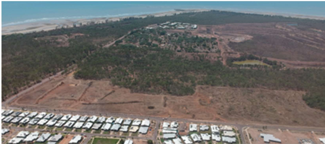
Lee Point peninsula with land clearing for Stage 1 in the foreground– photo Oct 2021
